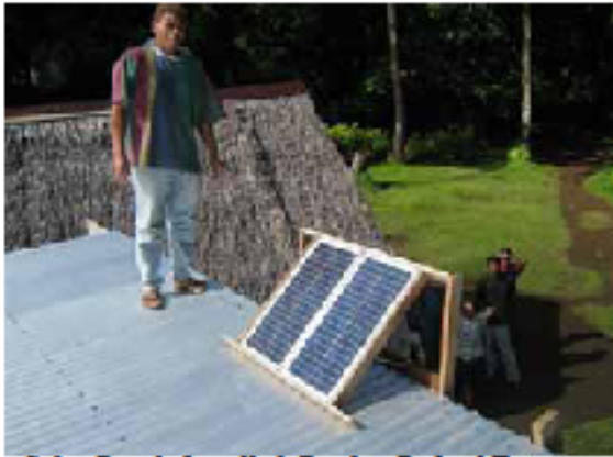
Solar Panels Installed. Brother Pethuel Tamga at Lombanga Village, West Ambae
